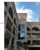
墨西哥蒙特雷FA中心 Mexico Monterrey FA Center Monterrey Office, Mitsubishi Electric Automation, Inc.
